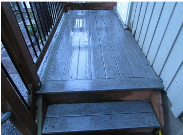
Deck & Stairs-Entry-Top Boards
