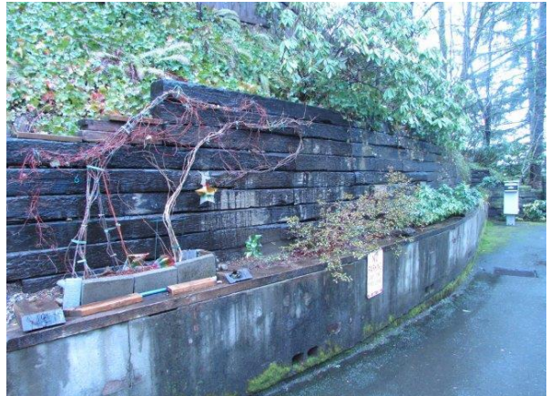
Wall-Retaining-Railroad Ties-Rock
