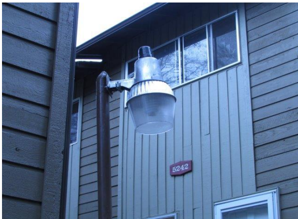
Lights-Exterior-Pole-Halogen-Head Only
